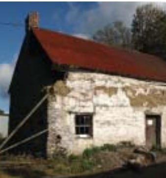
Above: Troedrhwiwallen before restoration work started (Tim Jones).
