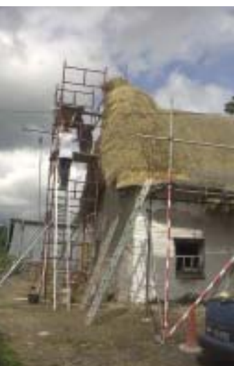
Above: Work in progress (Greg Stevenson).
