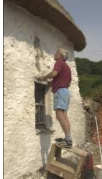
Above: Work in progress (Greg Stevenson).
